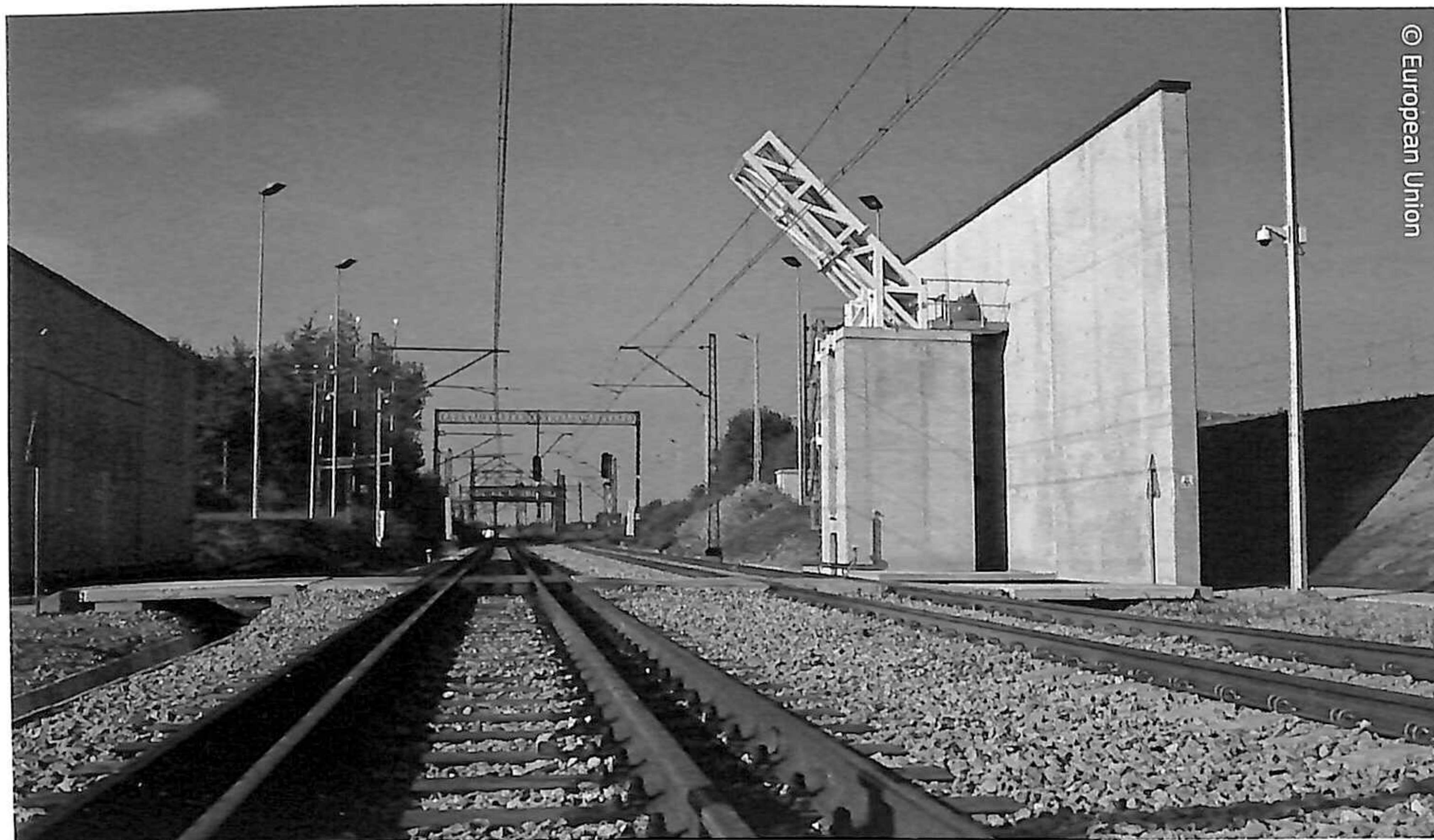
Checking wagons on railways: a train scanner at the border between Ukraine and Poland.
